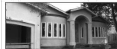
Saratoga. Brand New Single Story Home, 4BD/3BA, Office/Den, High Ceiling, Huge Master Suite. Price $1,895,000
